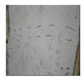
d) Transversal Crack in Control Slab
